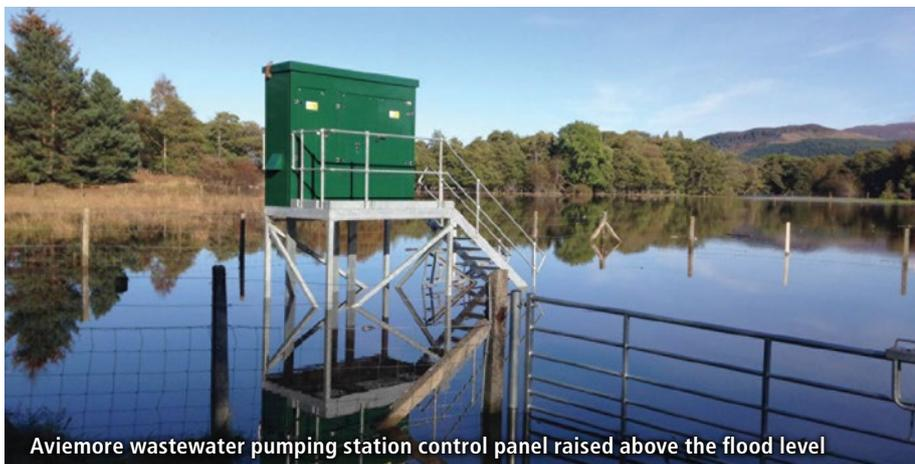
Aviemore wastewater pumping station control panel raised above the flood level
